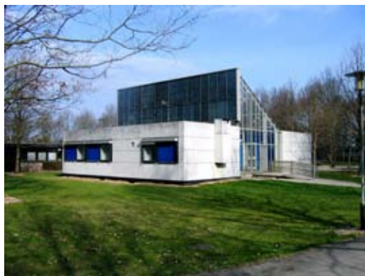
Figure 12. This is a photo of the “Null Energihuset” built at the Technical University of Denmark in 1975. It is the first house to attempt full seasonal solar heating through storage at a high latitude. Details are elaborated in the text. (Photo by author, April 2005.)
