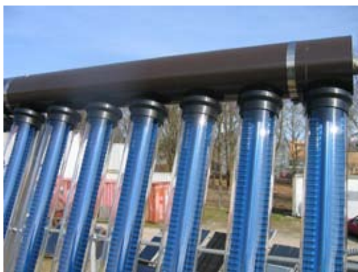
Figure 9. An evacuated glass tube with a heat pipe.
