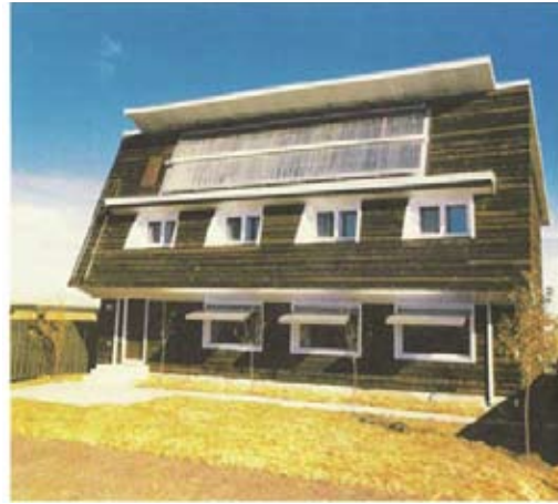
Figure 13. South side of the Saskatchewan Conservation House, 1977. Note the active solar panels (vacuum tube) on the upper part of the south wall, and the insulating shutters on the lower windows. An 11,000 liter water storage tank was incorporated to store solar heat within the house.
