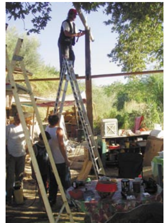
Building an outdoor kitchen.
